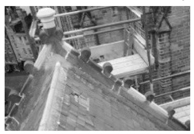
The west gable from above, after work had been completed: the lighter-coloured areas (including the top of the apex stone and the spaces between the third and fifth crockets on the right) are new stonework.
