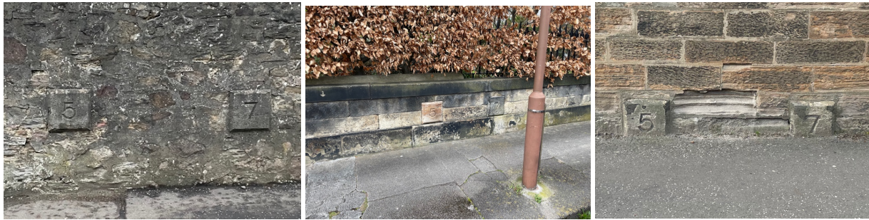
Stone markers in Canaan Lane, (Whitehouse Lane not shown), Hope Terrace, Strathearn Road.
